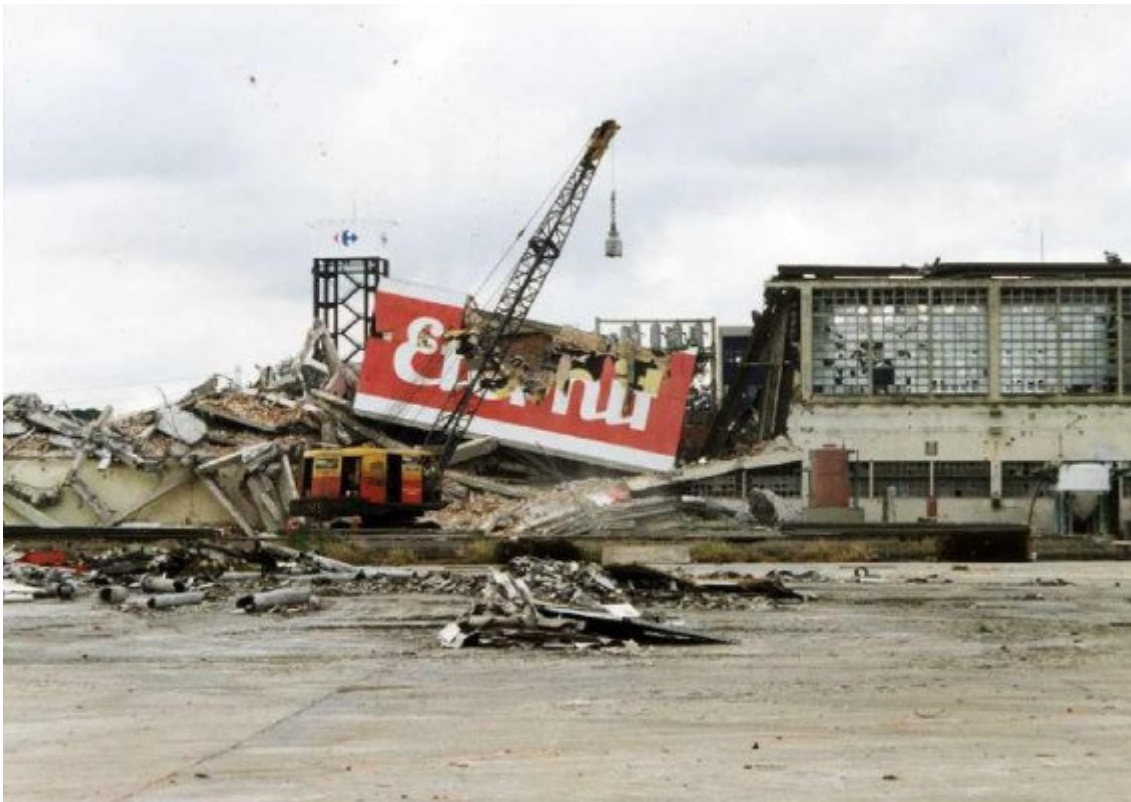
Demolition of the Osasco plant in 1995.
